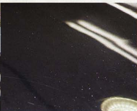
With the area washed clean and dried, the inspection process can begin. Adequate lighting is important so that every imperfection can be viewed. Notice how the reflection of the halogen light looks blurry? That's caused by orange peel. The process we will use to remove the scratches and swirls will also knock some of that down.
